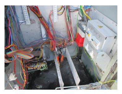
Where the NIE supply goes directly into an ITS controller cabinet, ITS providers should make it a <u>high priority</u> to instigate a programme of work to transfer the NIE cut-out to a separate supply mini pillar.
