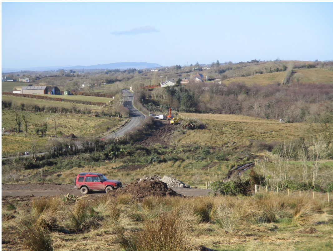
A32 Cornamuck site clearance works
