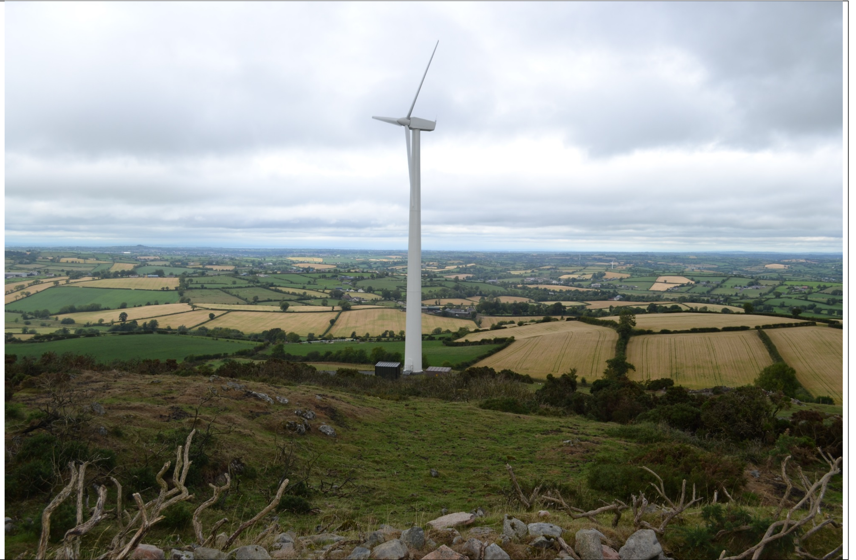
View from the cairn towards the turbine and electricity cabinets.
