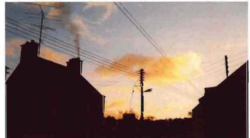
Wires before removal
