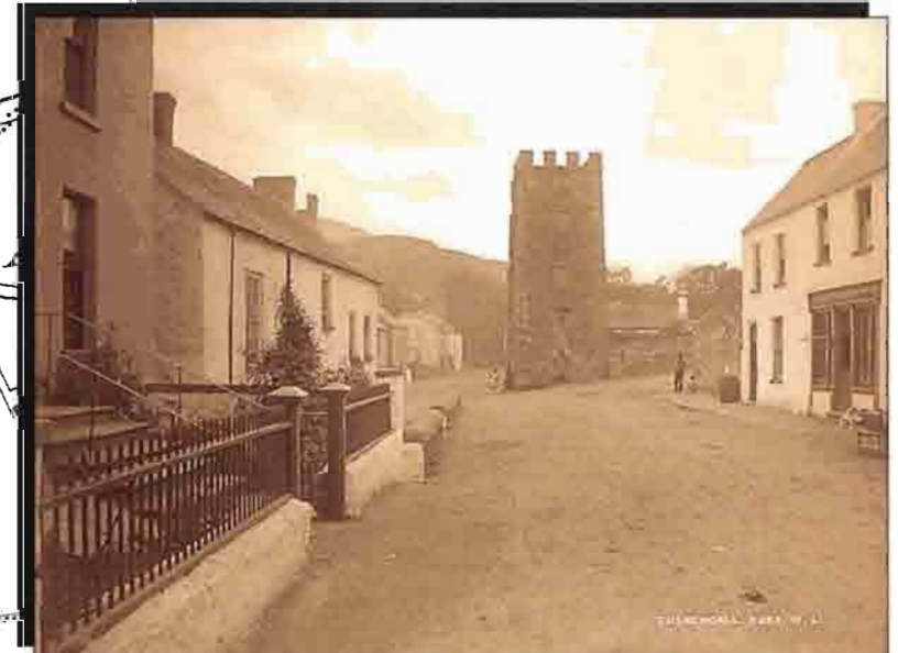
Curfew tower from shore st
