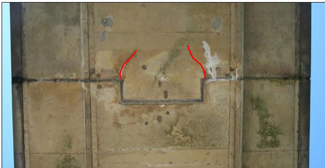
Figure 15: Fine cracks to half joint
