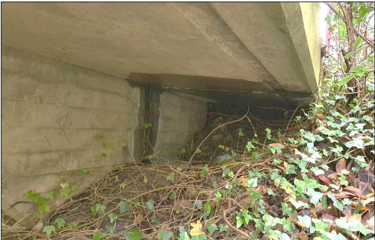
Figure 14: Active leakage at abutment joints – November 2021
