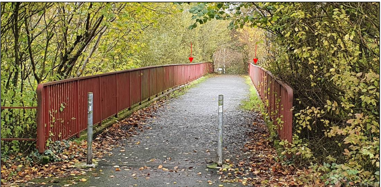
Figure 12: Overall view of parapets with visible deflection noted - November 2021
