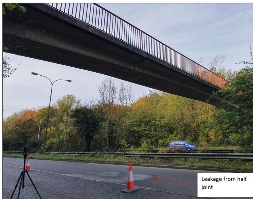
Figure 13: Active leakage from half-joint at Southbound carriageway
