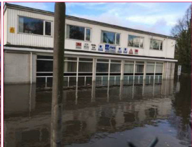
Figure 1 - Flooding at PWS, Greenbank Industrial Estate
