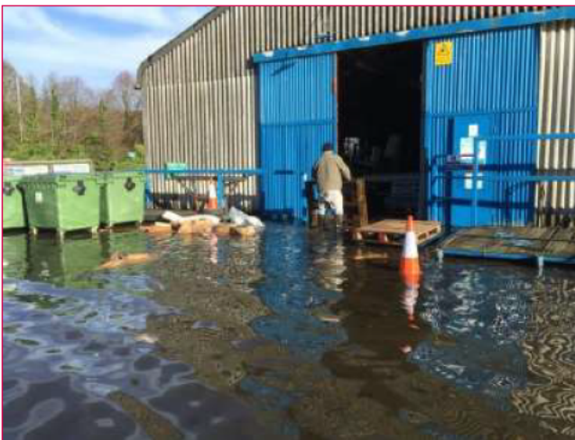
Figure 2 - Flooding at PWS, Greenbank Industrial Estate
