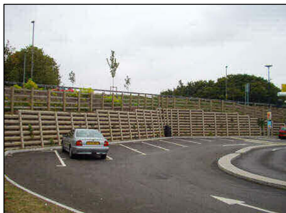
Plate 3.4 - Example of Retaining Structure
