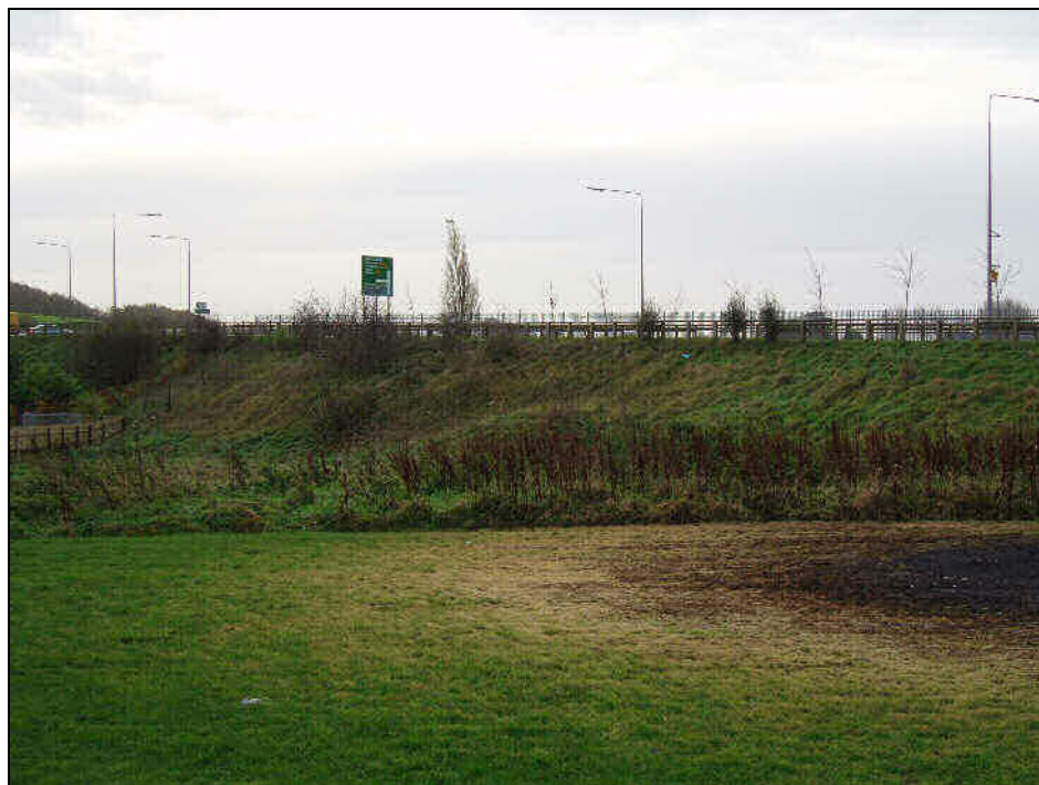
Plate 3.10 - View of embankment which carries the A28 south of Navan Street
