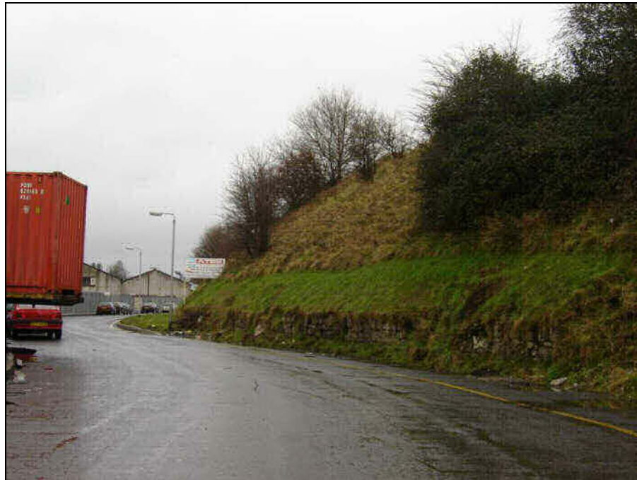
Plate 3.36 - Existing cuttings on Station Road
