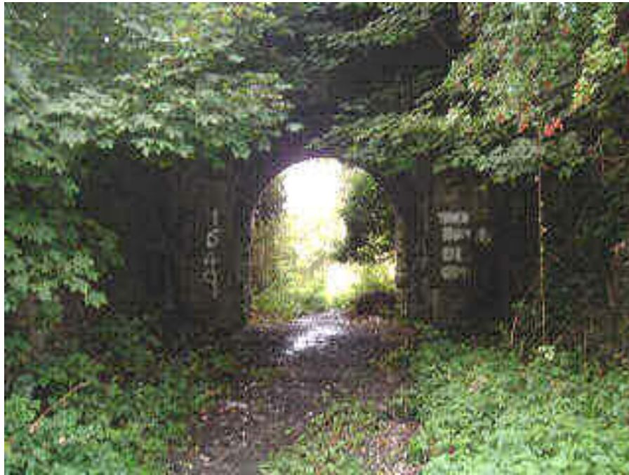
Plate 3.14 - Brick arch subway under railway embankment, near Ballynahone River
