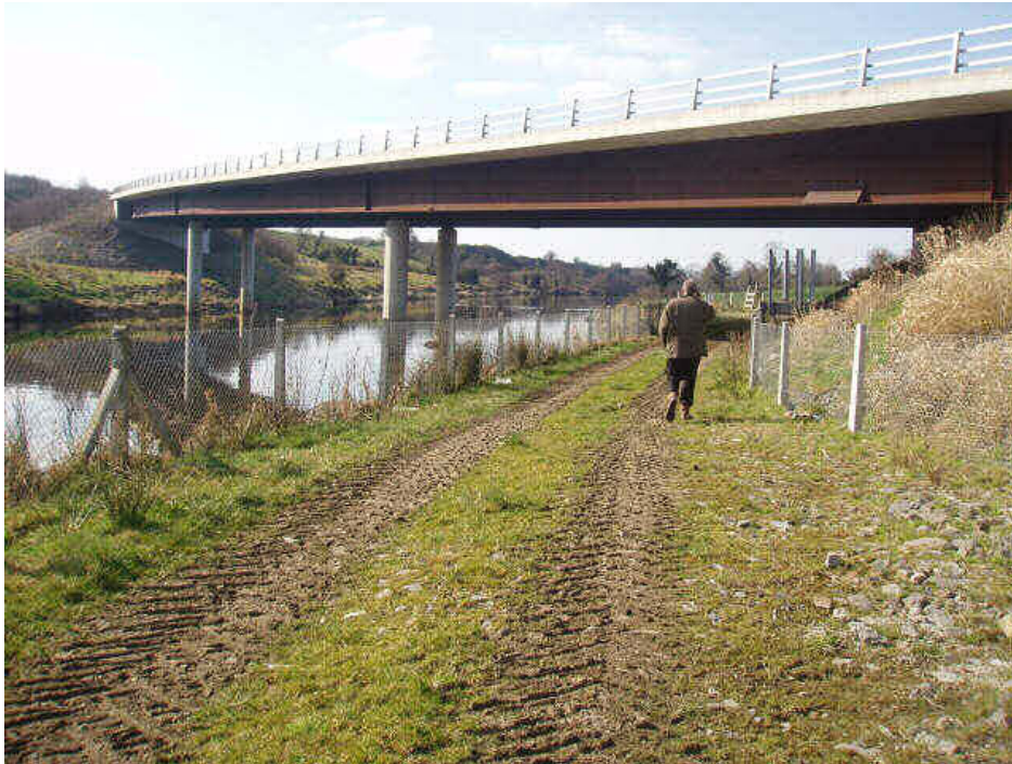
Plate 3.25 - Weathering steel bridge on Newtown Stewart Bypass
