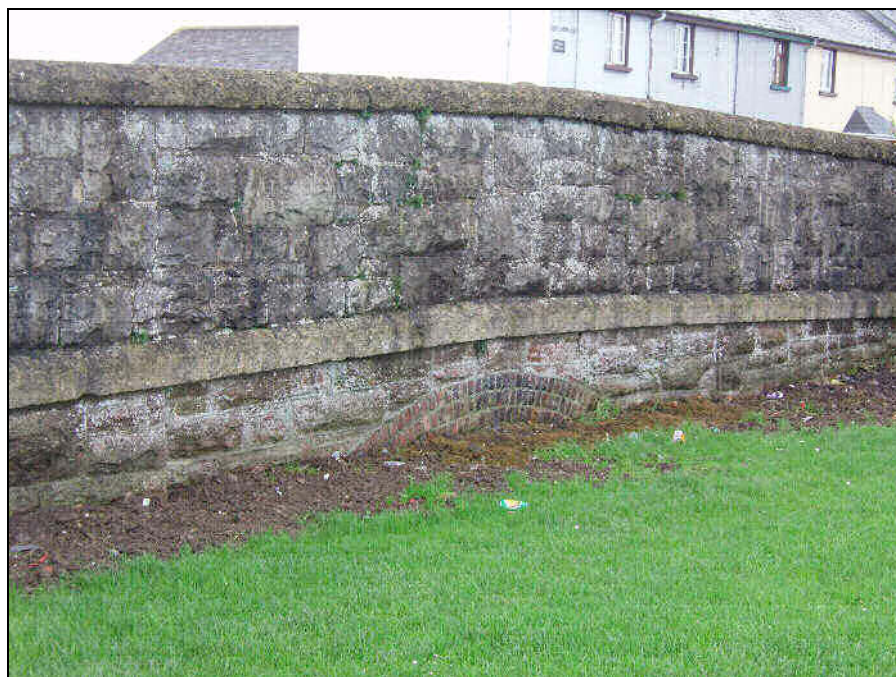
Plate 3.9 - Infilled masonry arch bridge at Navan Street
