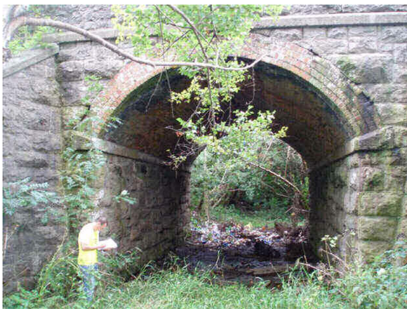
Plate 3.16 - Listed Masonry arch bridge conveying Cathedral road over disused railway cutting
