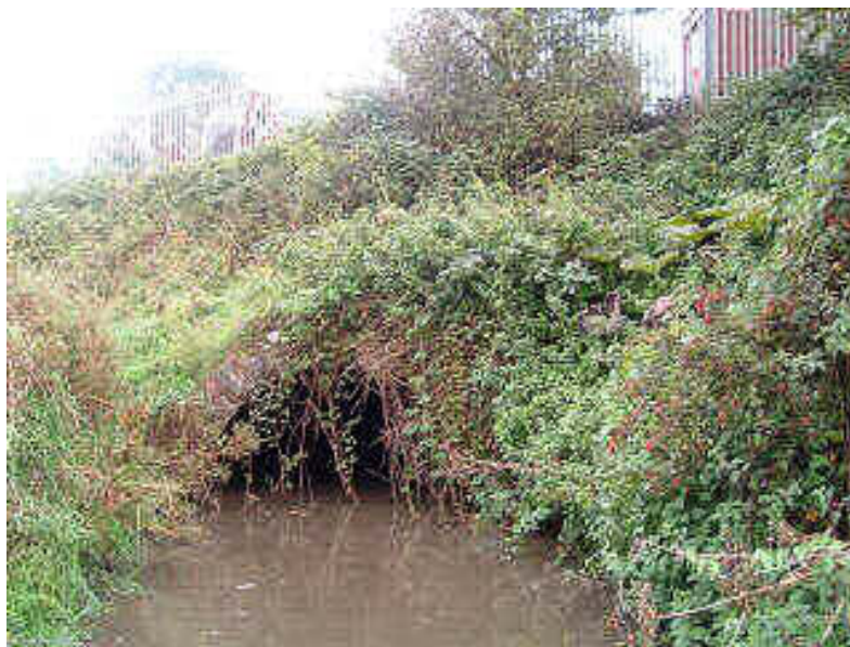
Plate 3.15 - Existing culvert at Ballynahone River
