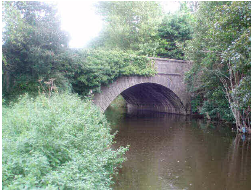
Plate 3.17 - Bridge conveying Killylea Road over River Callan
