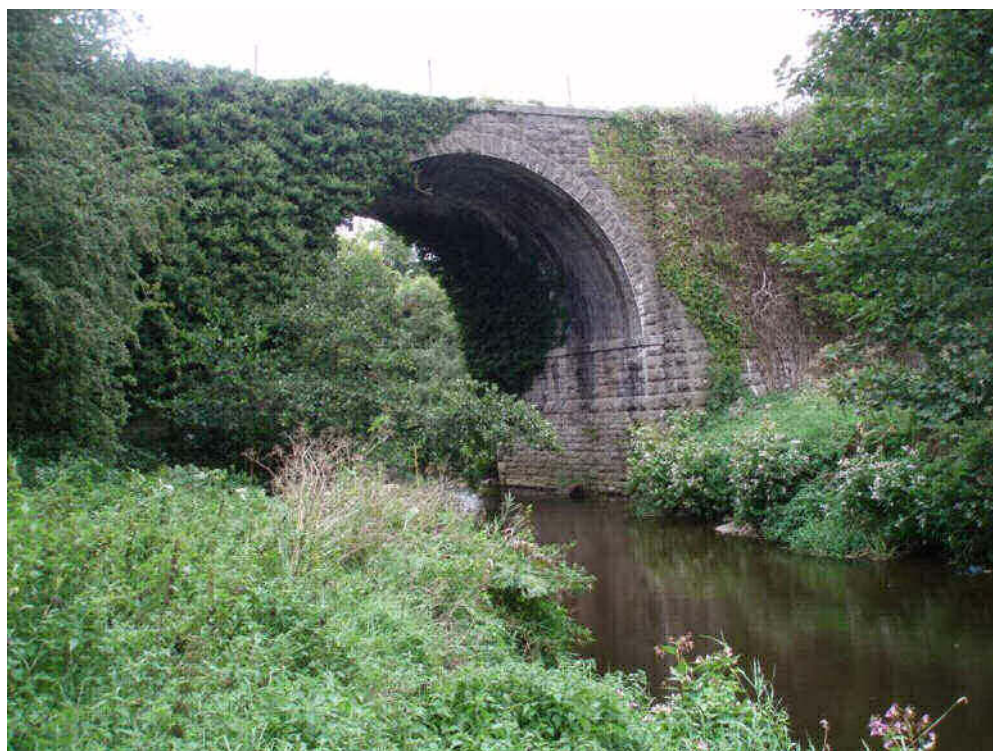
Plate 3.41 - Existing railway bridge near where the corridor crosses the River Callan.
