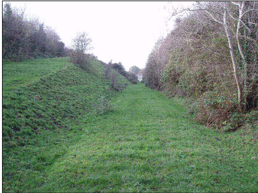
Plate 3.1 - Disused railway cuttings between Station Road and Mullinure Lane
