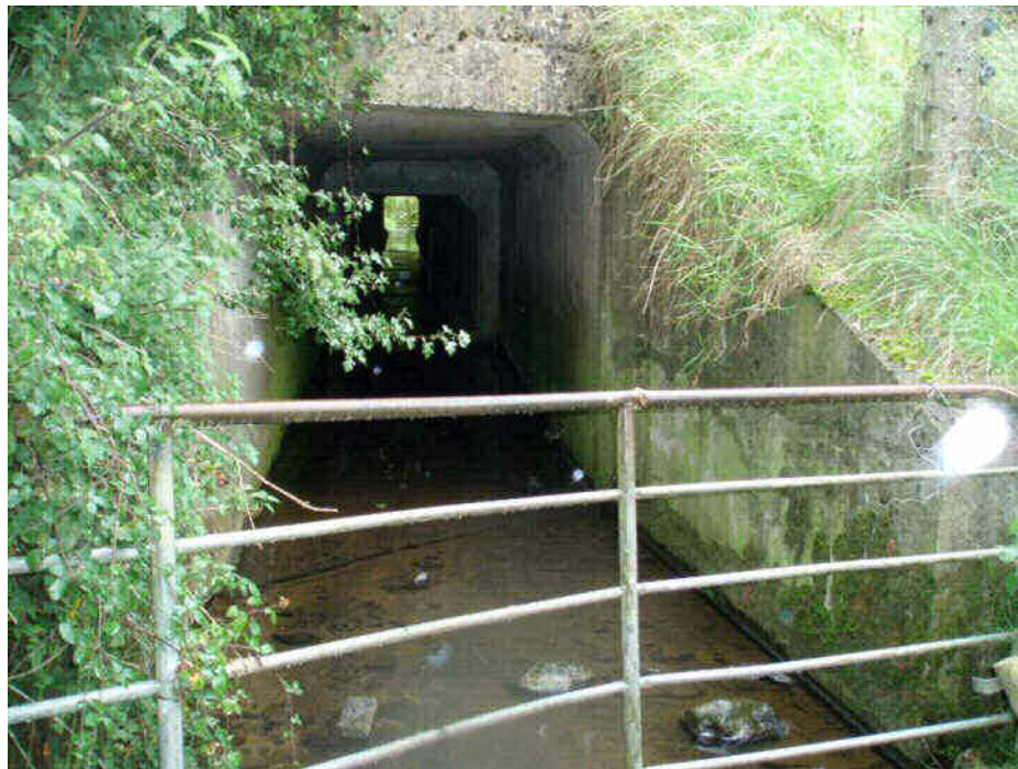
Plate 3.12 - Existing culvert under Moy Road: Route Corridor 3 crosses this stream
