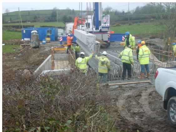
Lifting in of an edge beam
