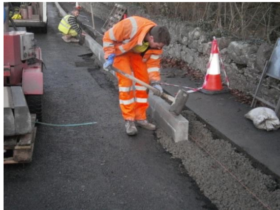
Adjusting the height of the newly laid kerb
