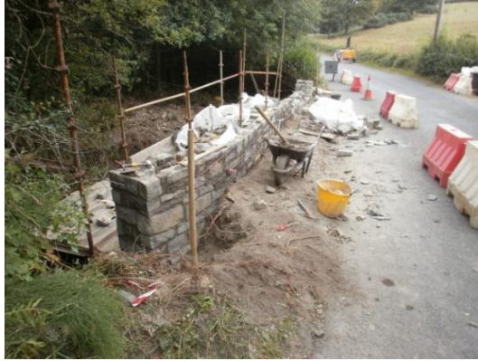
The parapet under re-construction
