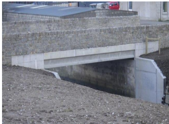
View from the West pier – Bridge complete
