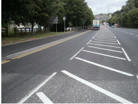
The start of the resurfaced section
