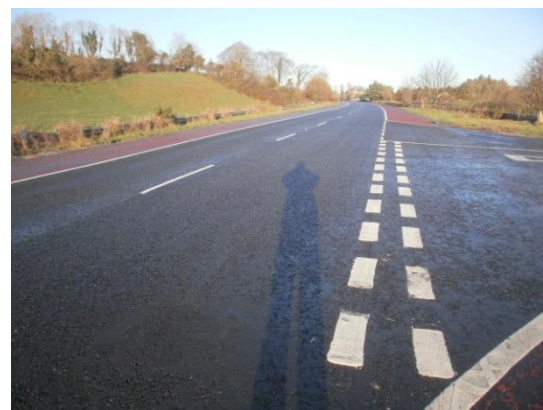
The start of the resurfaced stretch of road
