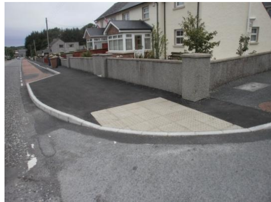
The start of one of the new stretches of footway
