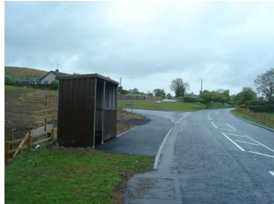
The junction at the end of works
