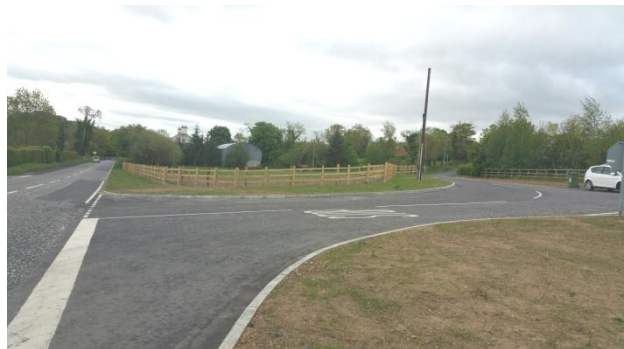
The new junction showing the improved sightline.
