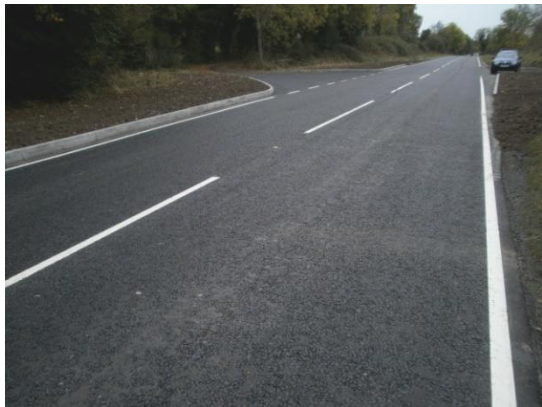
A section of the Monaghan Road after resurfacing
