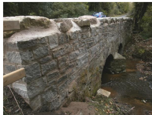
The cut water after re-facing works
