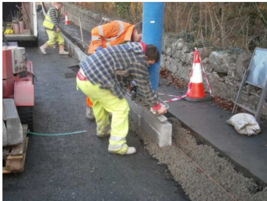
Laying new kerbs along the road edge
