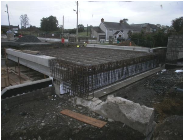
Works at the site to replace the bridge decking.
