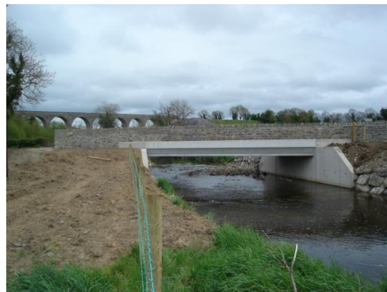
View of completed Bridge
