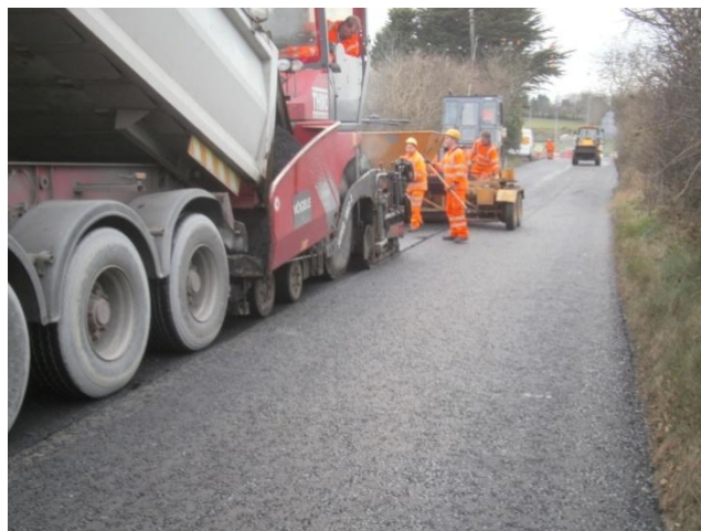
Asphalt resurfacing being carried out within the Division
