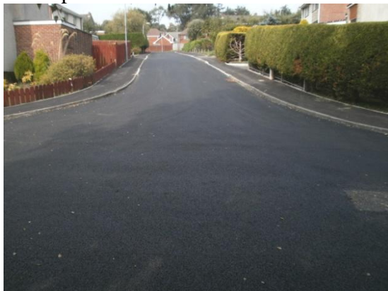
At the top end of the estate after resurfacing
