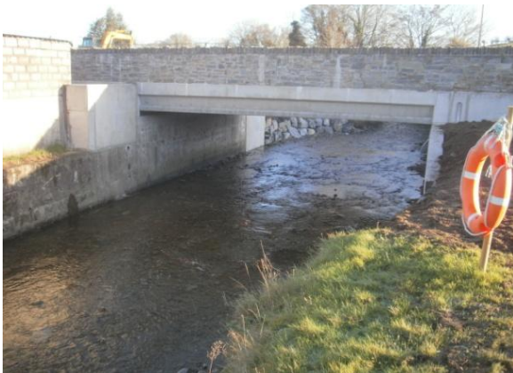
The rear of the East pier
