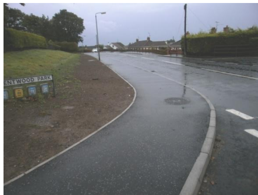
The junction at the completion of the works
