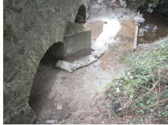
A view of the cut water during re-construction
