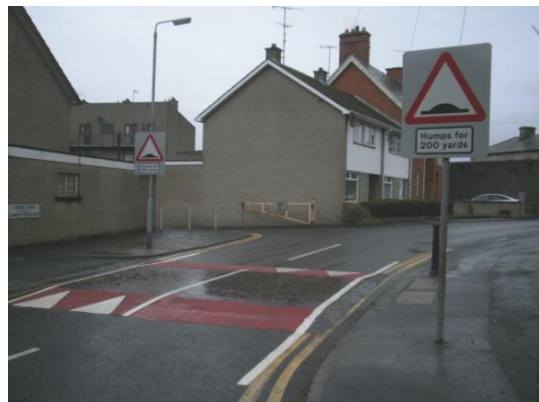
Sign and hump at the start of the scheme
