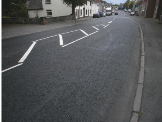
Main Street after resurfacing works
