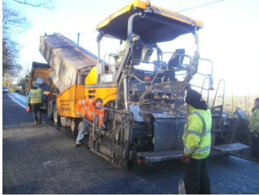
The start of asphalt laying
