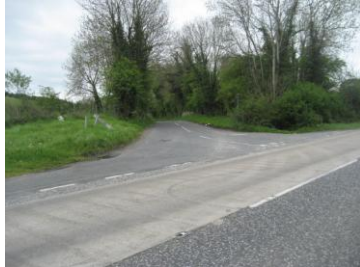
At the start of works
