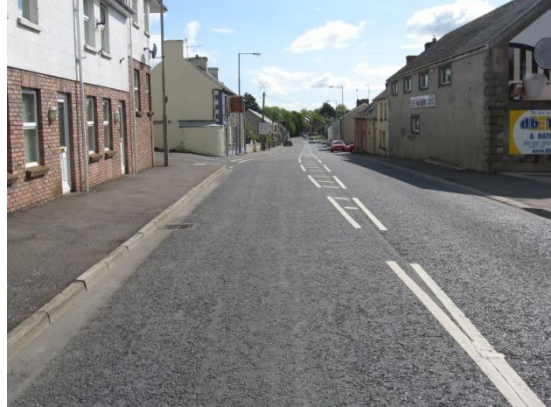
The road following resurfacing
