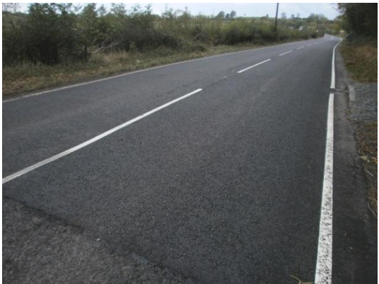
The start of the works on the Monaghan Road
