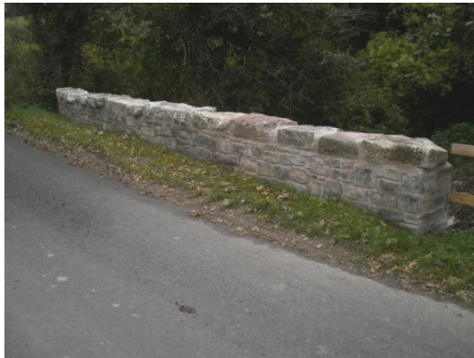
The parapet at the completion of works
