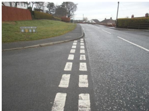
The view prior to works at the junction
