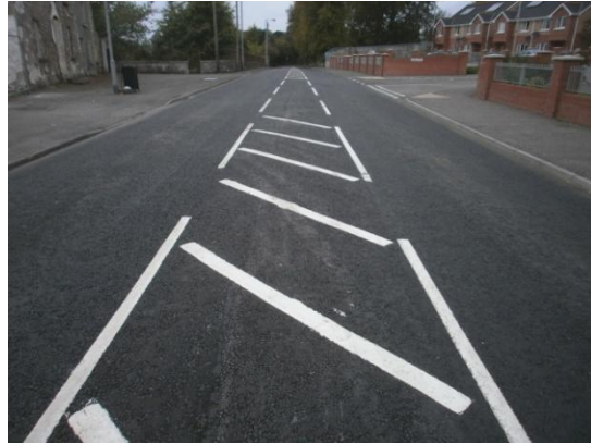
Another view of Main Street after resurfacing
