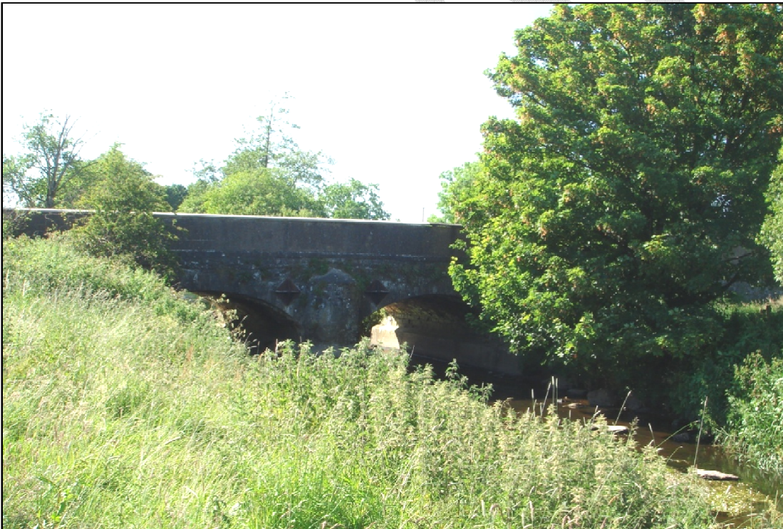
Photograph 2.1 – Existing Shannaragh Bridge
