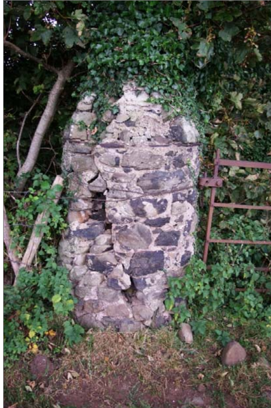
Plate 27: Blue Route: Coursed masonry gate pier at entrance to derelict dwelling (Plate 26) – to the west.
