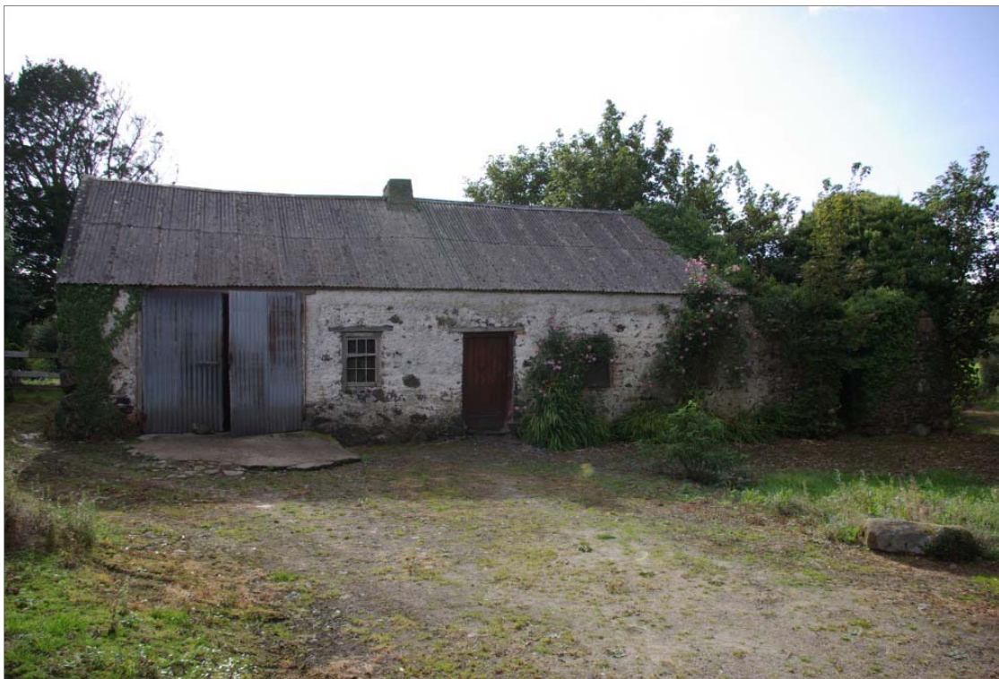
Plate 20: Pink/Purple Routes: two-bay single storey vernacular structure (Tommy Martin's cottage) north of Pink Route east of Killyfaddy Road and Flax Mill site at Leckagh.
