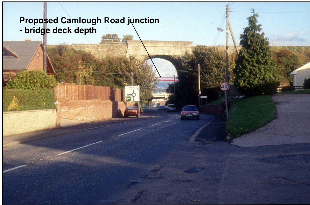
VIEWPOINT 06 - LOCATION OF PROPOSED CAMLOUGH ROAD JUNCTION AS SEEN THROUGH EGYPTIAN ARCH
