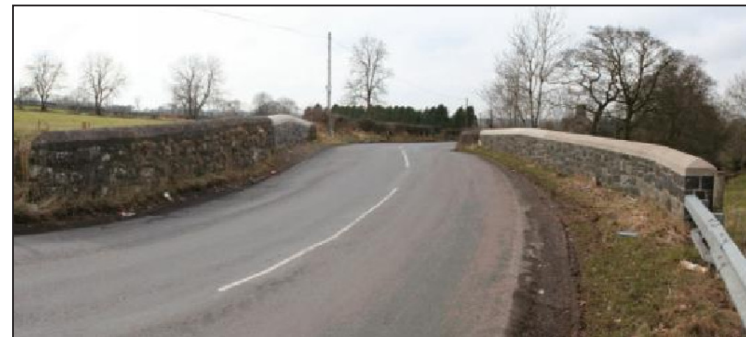
Date: 03/03/2010 Time: 15:10 X: 145236 Y: 549319 View Direction: 090° Height: 91m AOD
