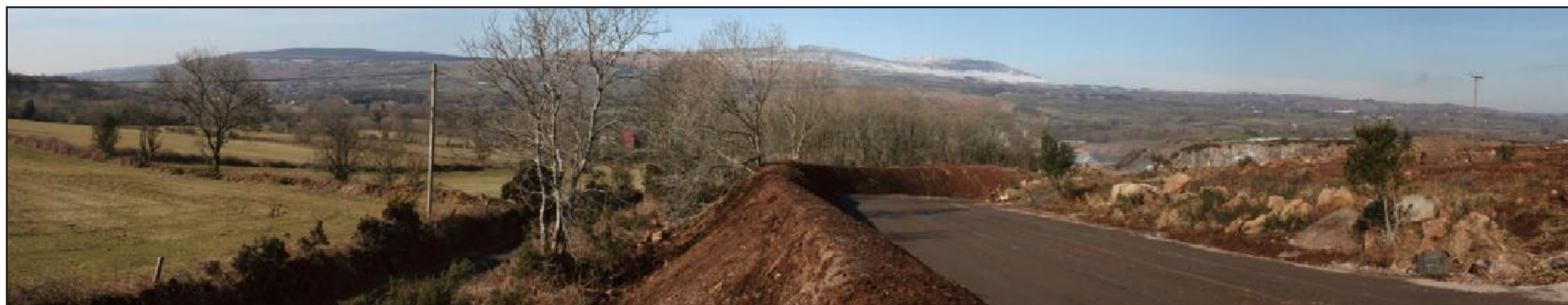
Date: 04/03/2010 Time: 14:39 X: 140282 Y: 543034 View Direction: 270° Height: 148m AOD
