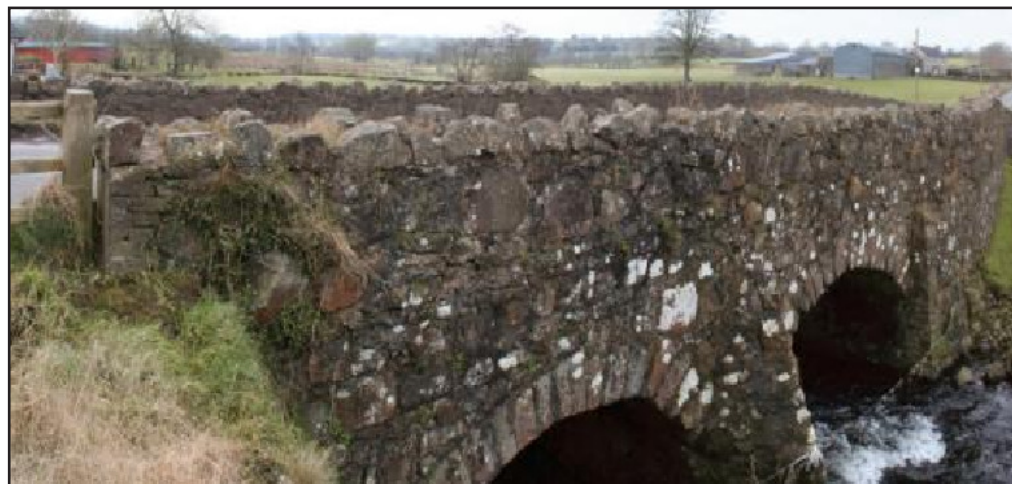
Date: 03/03/2010 Time: 14:57 X: 144799 Y: 549374 View Direction: 270° Height: 84m AOD
