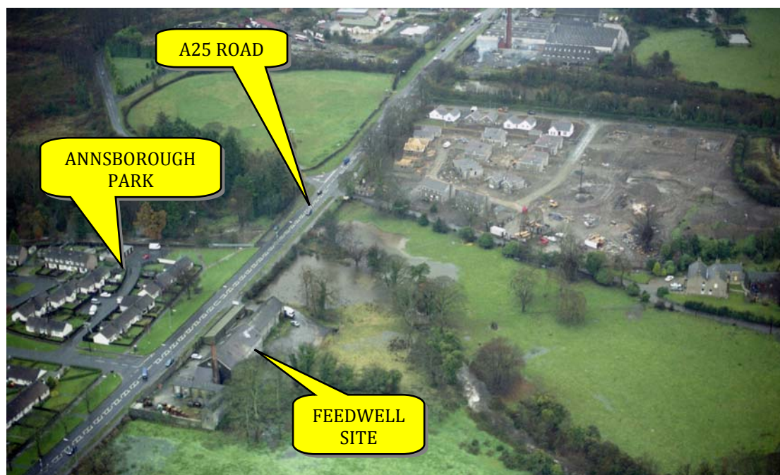
Fig. 3.2 – Aerial photograph post November 1997 Flood Event.
