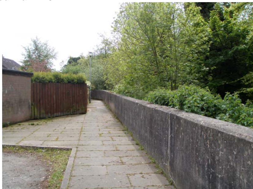
Fig. 4.7 – Designated Flood Wall
