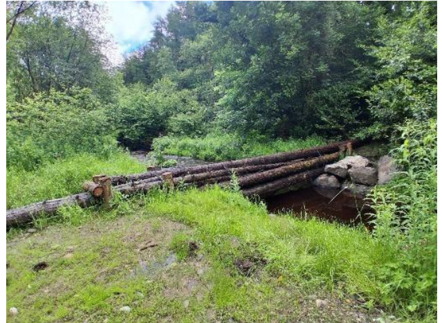
Timber structures extending into the woodland floodplain.
