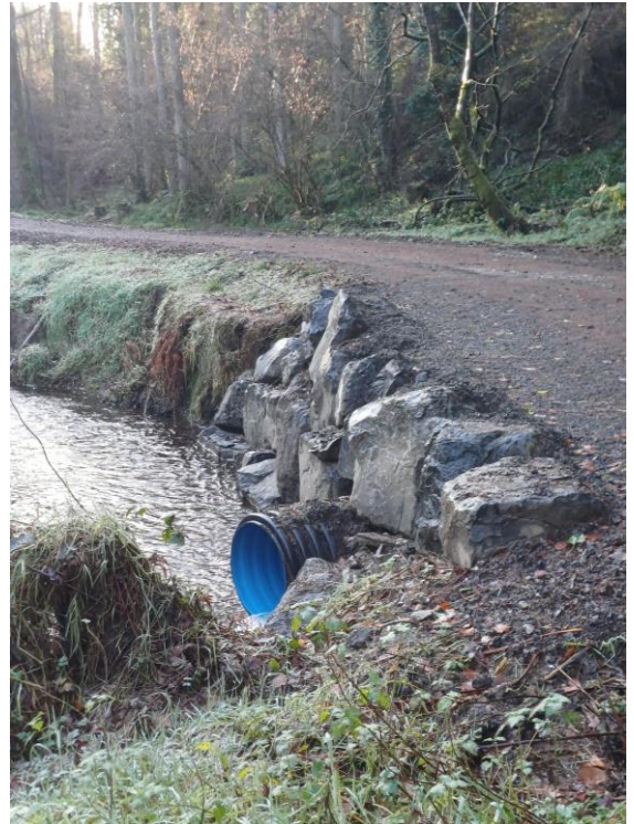
Riverbank works within the forest has helped stabilise eroded banks, enhancing fishery habitat
