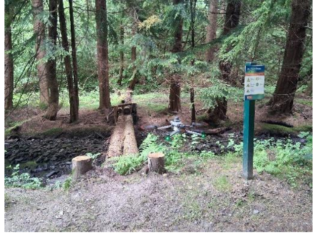
Safety signage at a dam location
