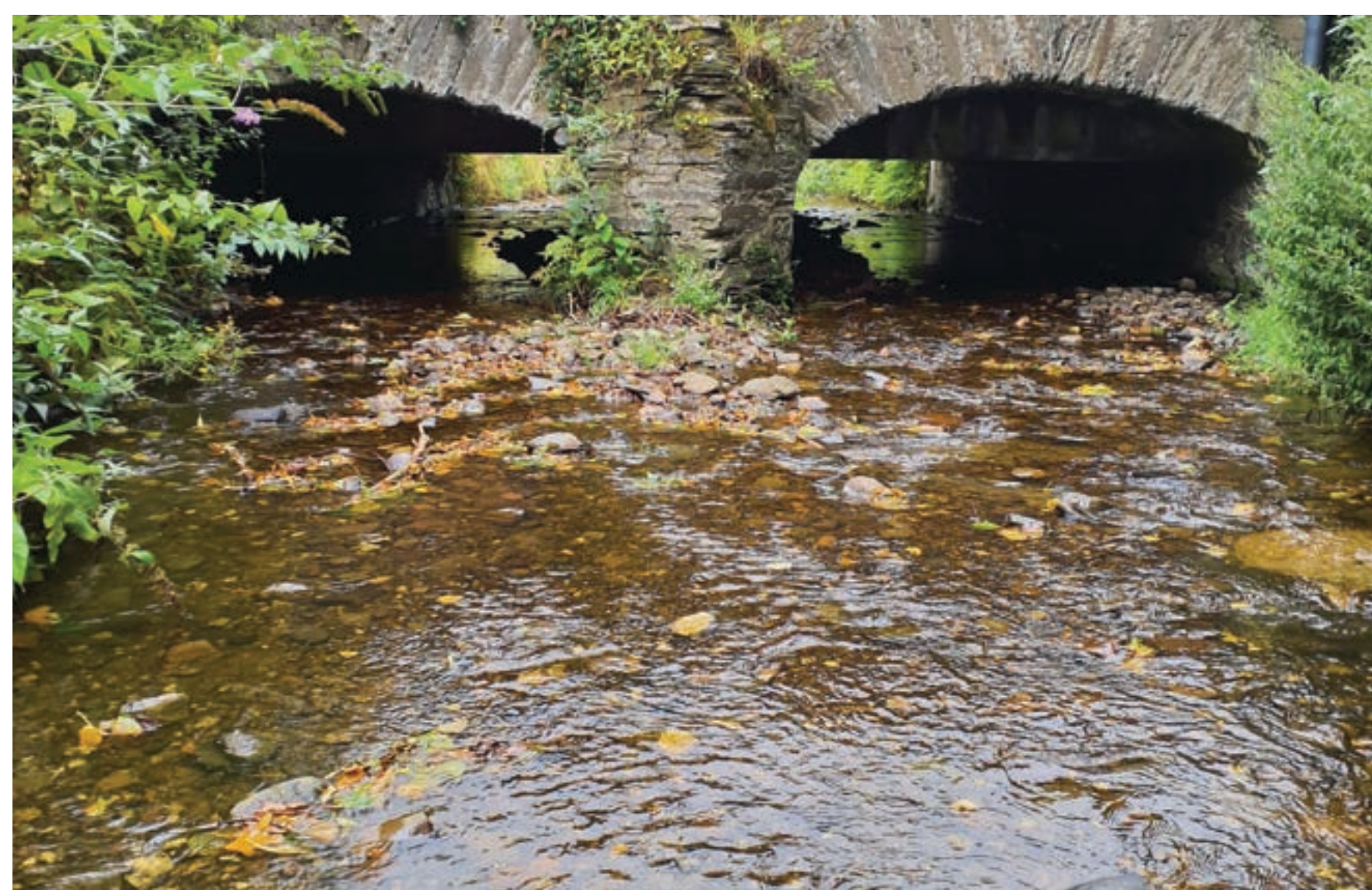
Watercourse maintenance and clearance of blockages on the Muff and Castle Rivers.
