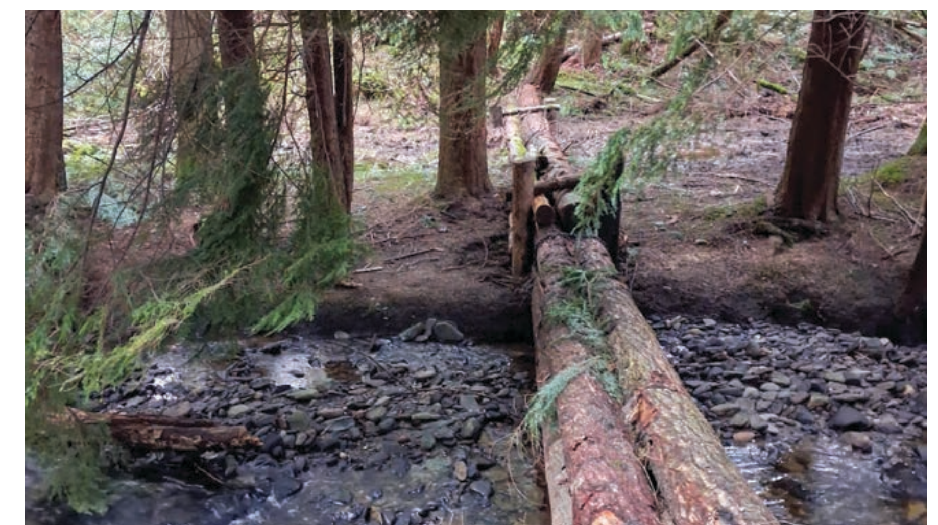
Nature based Solutions, installed no. 10 Leaky Dams at Muff Glen Forest to augment the proposed scheme.
