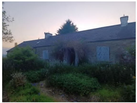
South Elevation of Pollan Rua Cottage Annexe
