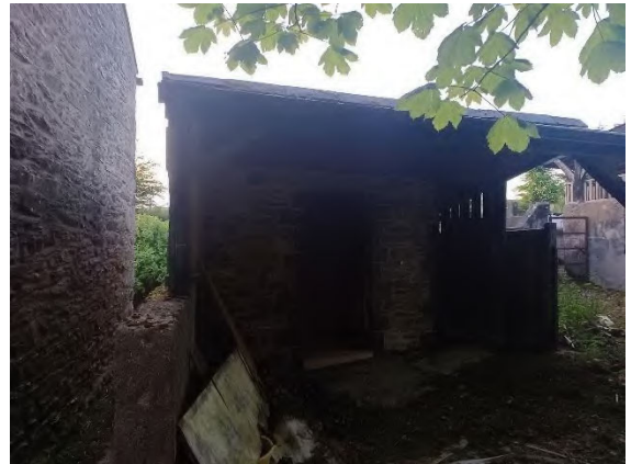
South Elevation of Boiler Shed
