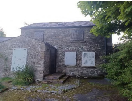
South Elevation of Main Pollan Rua Cottage
