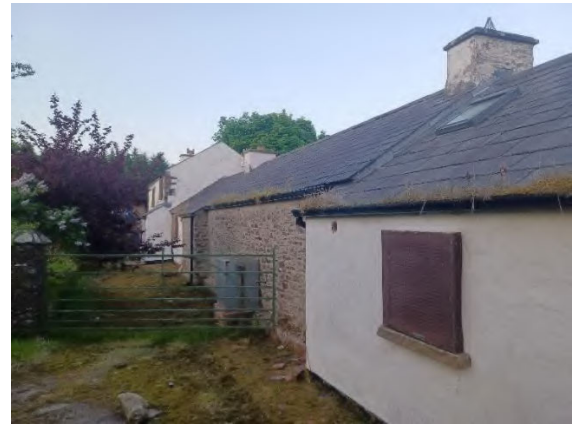
North Elevation of Pollan Rua Cottage Annexe
