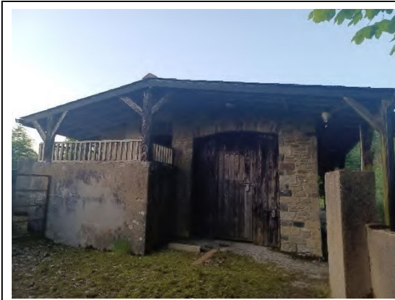
West Elevation of Livestock Shed
