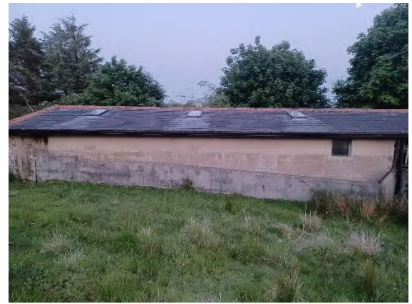
North Elevation of Livestock Shed
