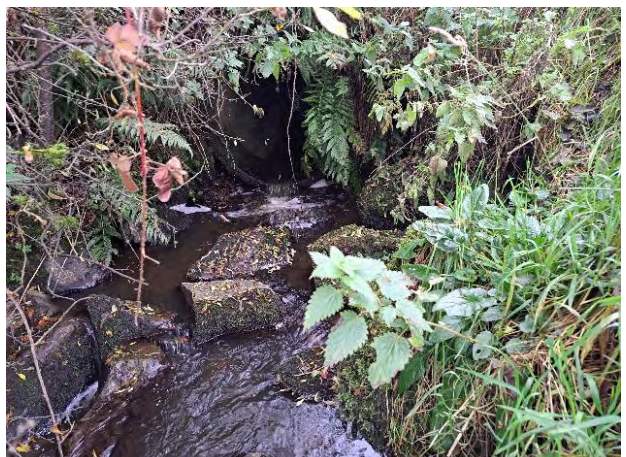
Pipe culvert Downstream End
