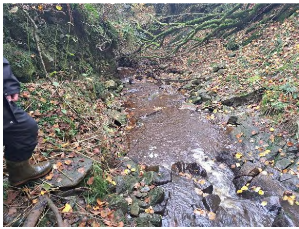
Chute Looking Downstream
