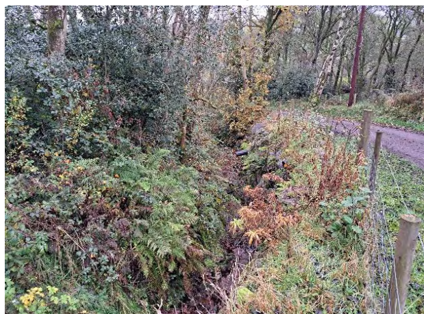
Road Culvert Looking Downstream
