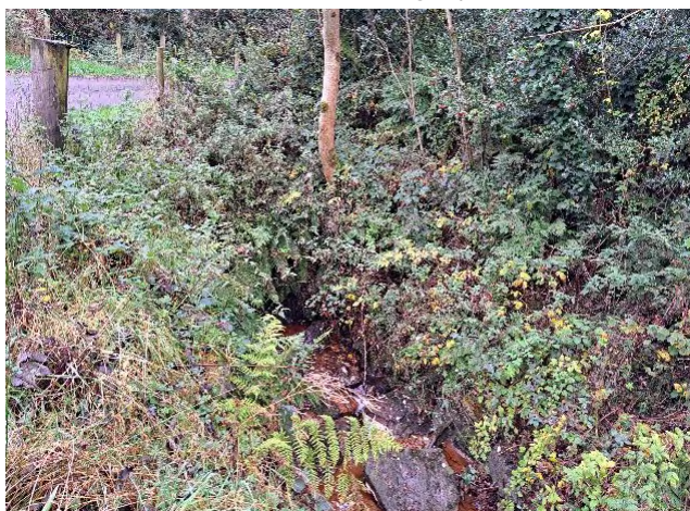
Road Culvert Looking Upstream
