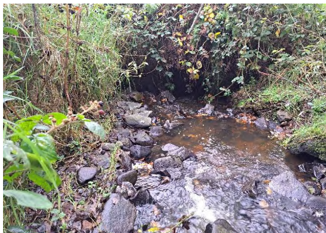
Pipe culvert Upstream End
