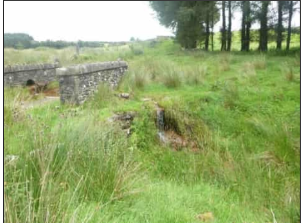
Photograph 6: Ford and culvert at downstream end of reach
