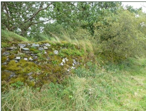
Photograph 3: Bank flood protection wall (land side)
