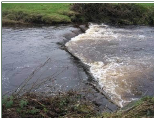
Photograph 3: Channel bank protection and ford access with Himalayan balsam invasive species
