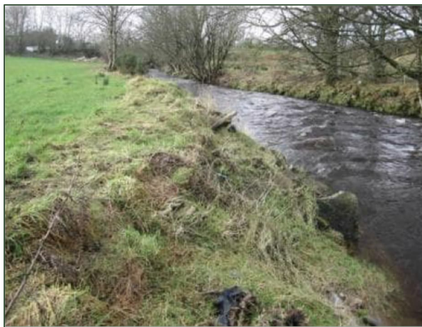
Photograph 4: Channel bank and riparian landuse
