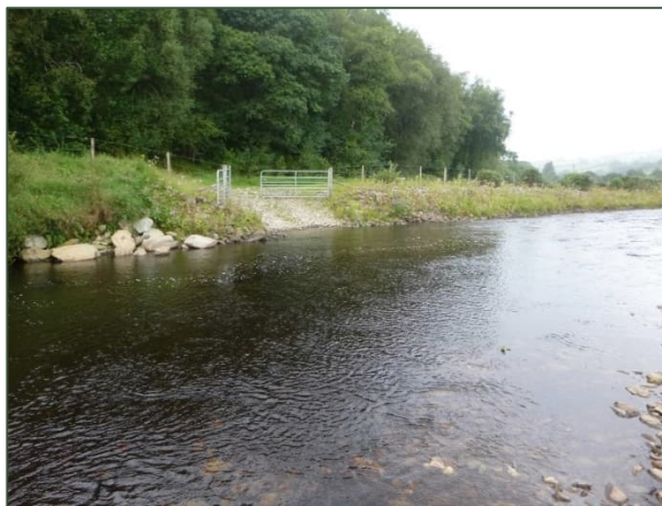
Photograph 3: Channel bank protection and ford access with Himalayan balsam invasive species
