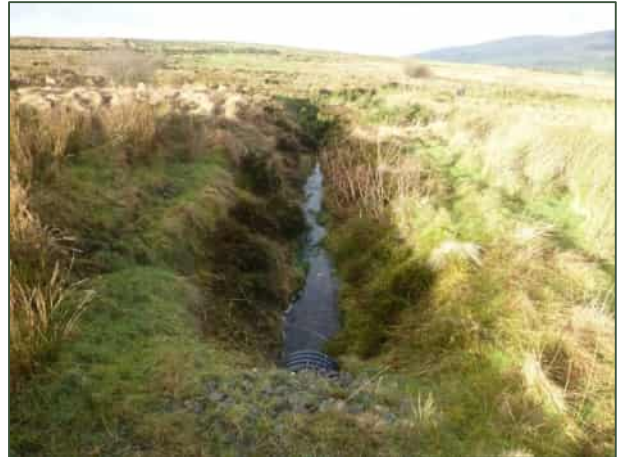
Photograph 4: Straightened section of burn channel with small, piped culvert
