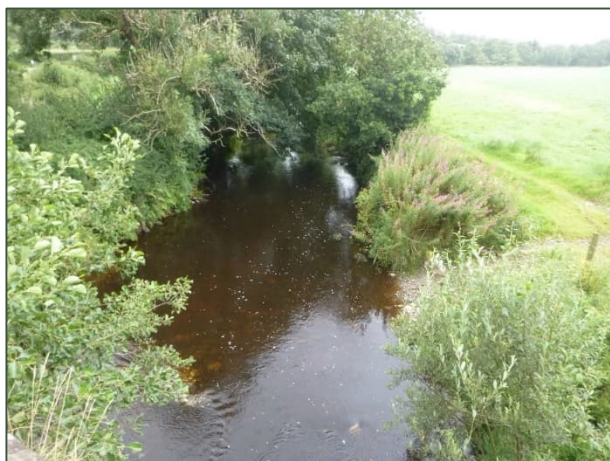
Photograph 1: Channel alignment at Drumlea Br. with floodplain on RHB
