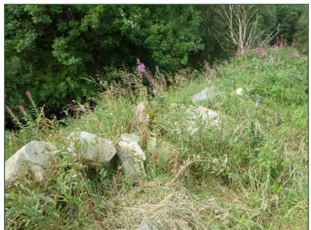
Photograph 4: Bank top with placed material for flood protection
