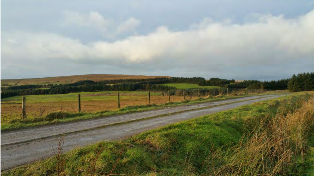
North section of the existing road to be abandoned (1)
