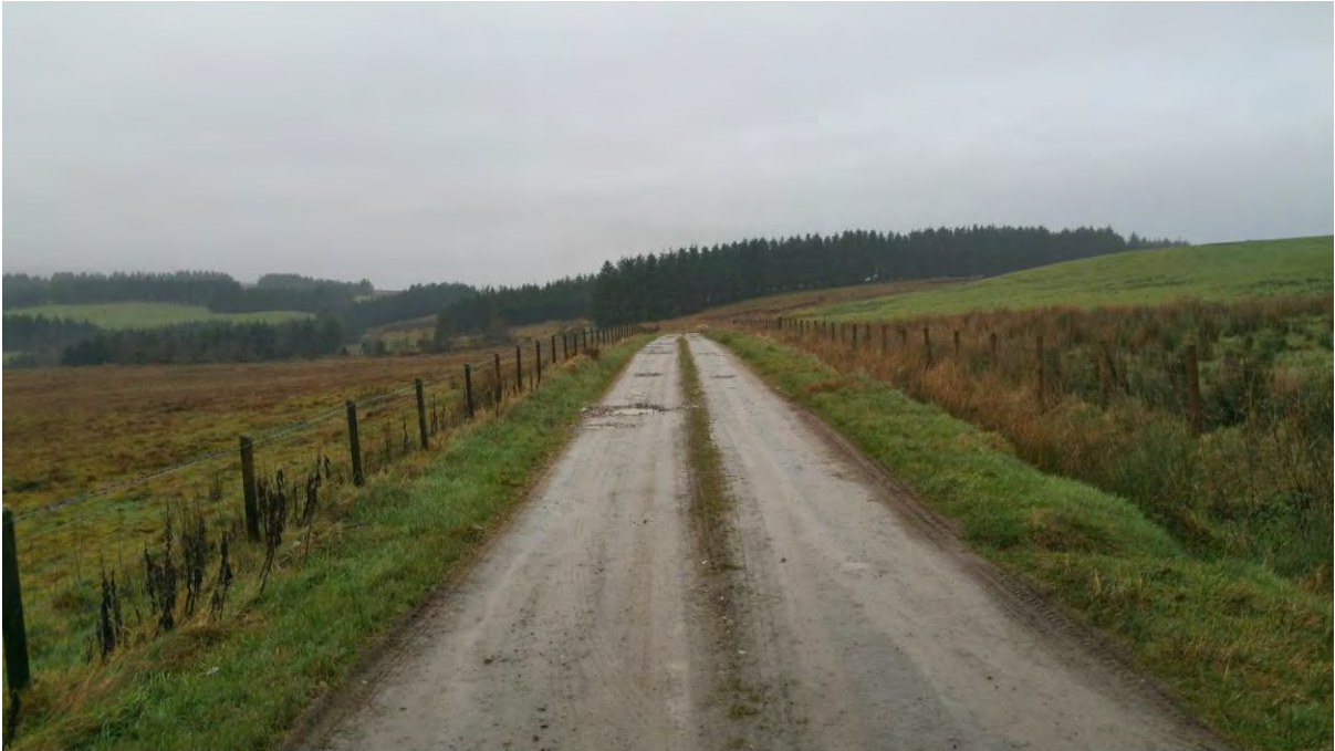
North section of the existing road to be abandoned (3)
